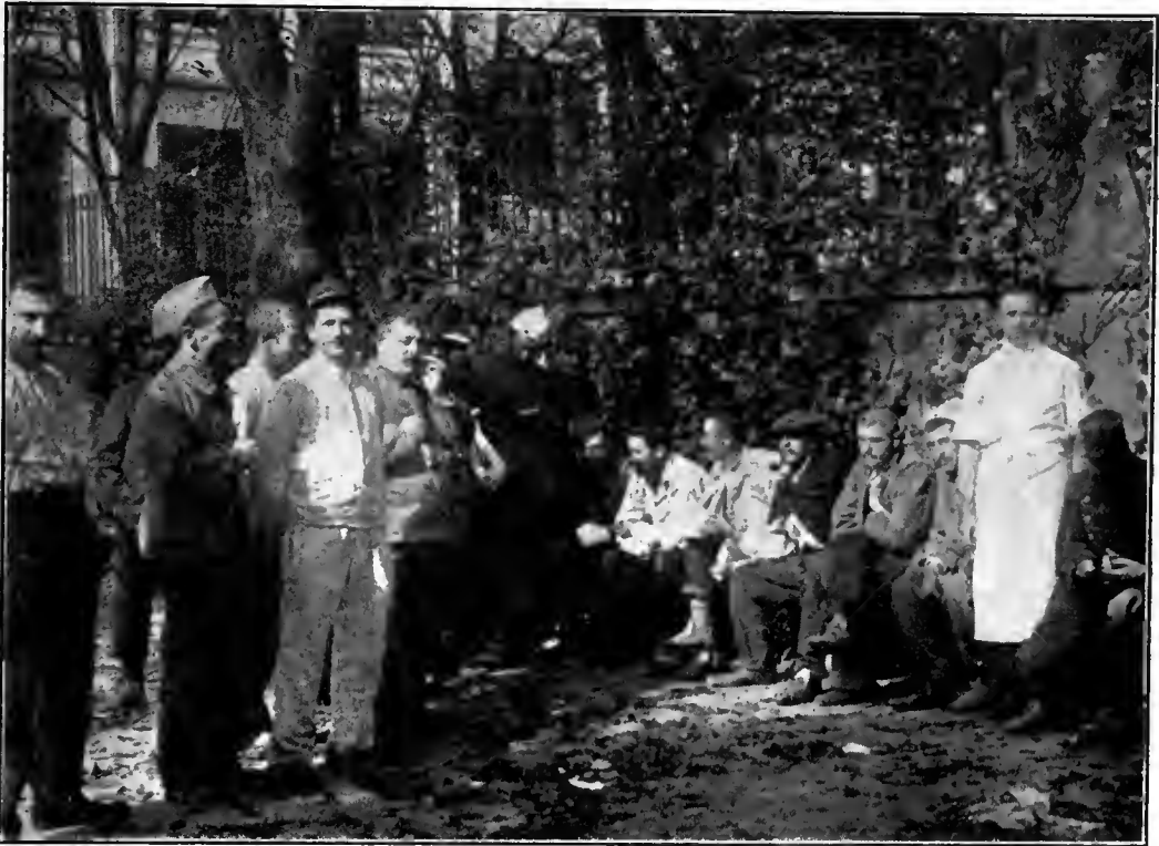
THE HOSPITAL AT VAL DE GRAS.
